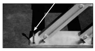
Fit handrail in correct position and securely fasten to the Stair Unit. Ensure bolts are tightened.
